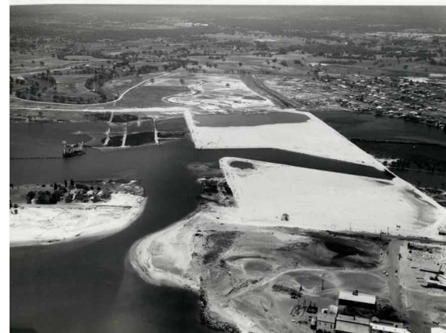
Picture 4: Inner Harbour Dredging, 1970.
