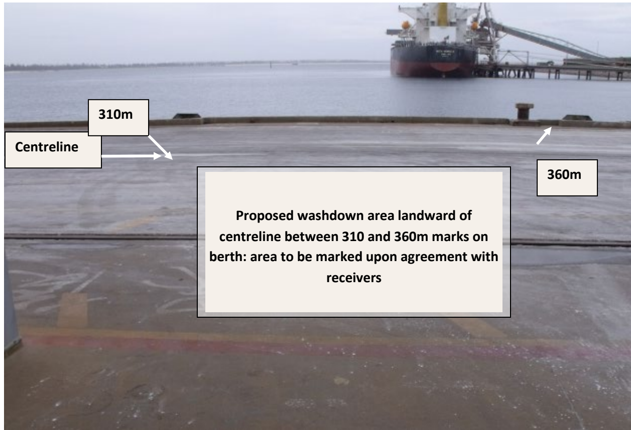
Figure 6. Alignment of hopper washdown between 310 to 360m mark on berth 2, landward of berth centreline. The area seaward of centreline should be kept clear to allow cleaning contractor to sweep up any spills from the containment used to capture hopper washings. Ensure all services lids are sealed in this area.
