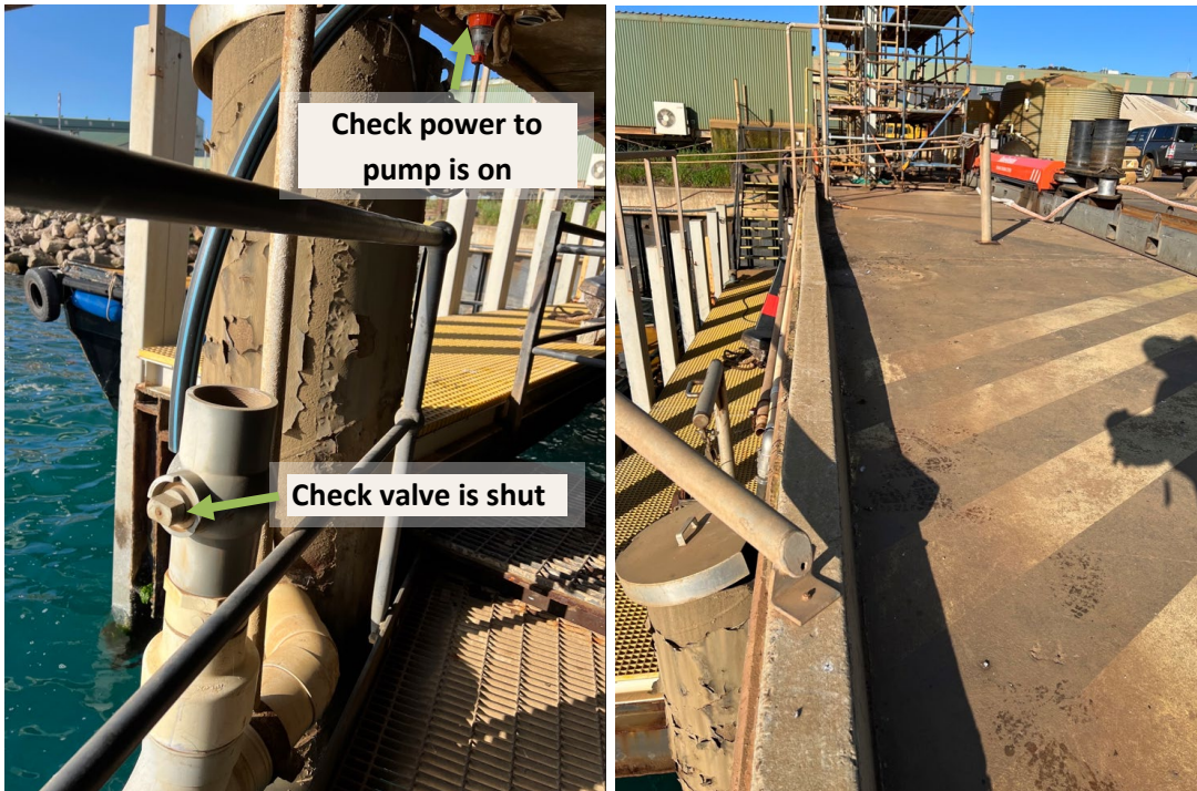
Figure 2 Berth outlet valve shown in closed position to divert water to tanks
