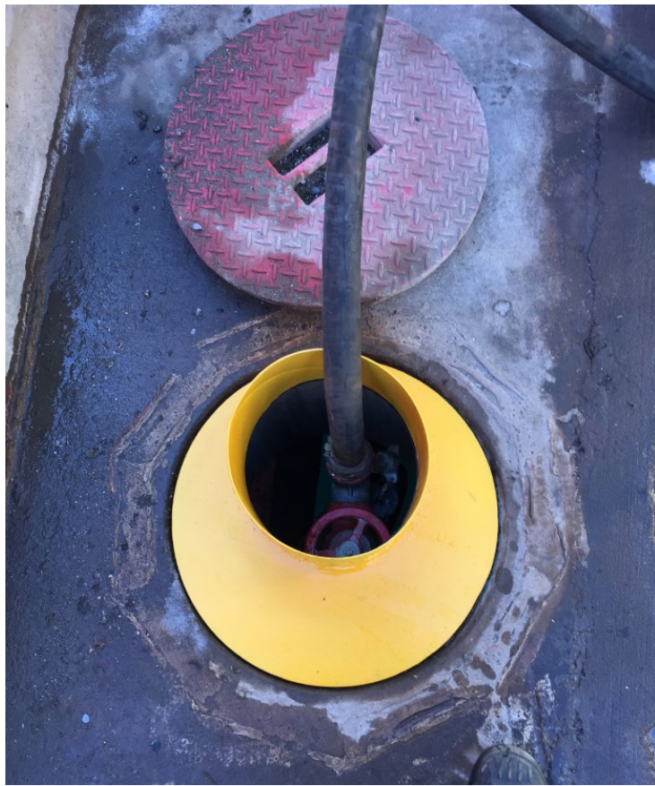
Figure 8. The modified hatch cover to minimise fertiliser washwaters entering ocean when using the hose.
