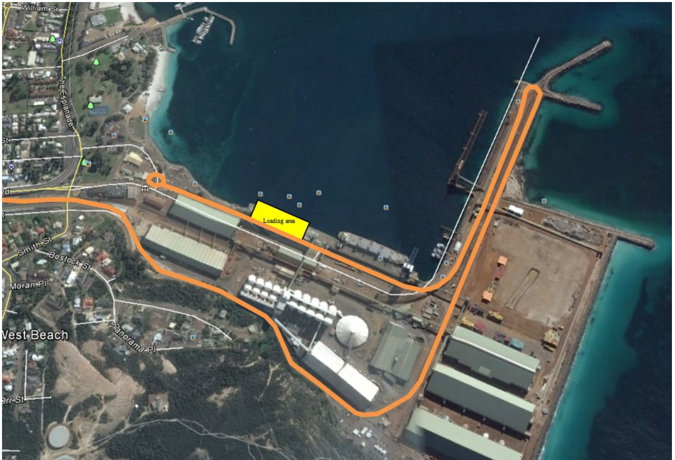
Figure 2. Route (orange line) to be swept by stevedore commissioning a cleaning contractor on truck routes to and from Berth 1 loading areas (in yellow).
